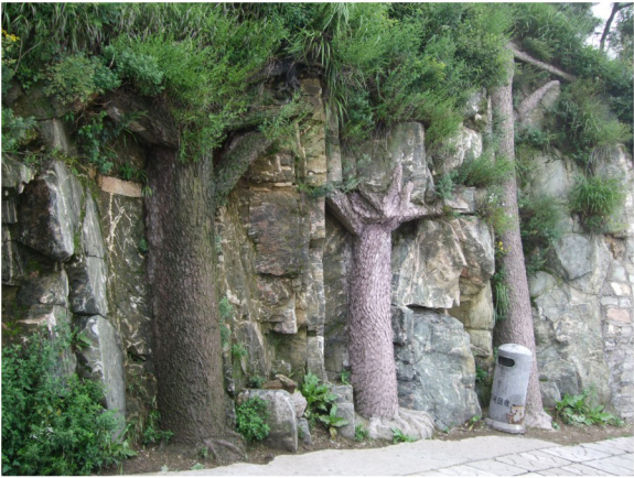
图5 危岩树干型支撑 Fig. 5 Trunk-like support structure for perilous rock
