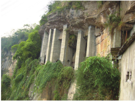
图4 万州太白公园危岩支撑结构 Fig. 4 Support structure of perilous rock at Taibaiyan, Wanzhou
